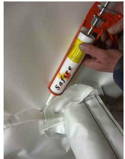
Left: Multi-Collar fitted to an insulated service penetration. Note how the collar encloses the wrapped service. Note the stapled overlaps and pleats on the main curtain.
